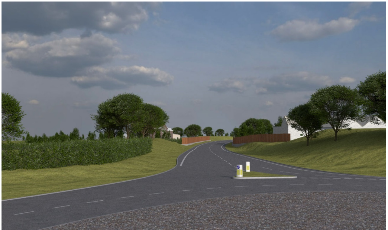
Earth bunds and noise barriers along proposed A737 adjacent to Barrmill Road
