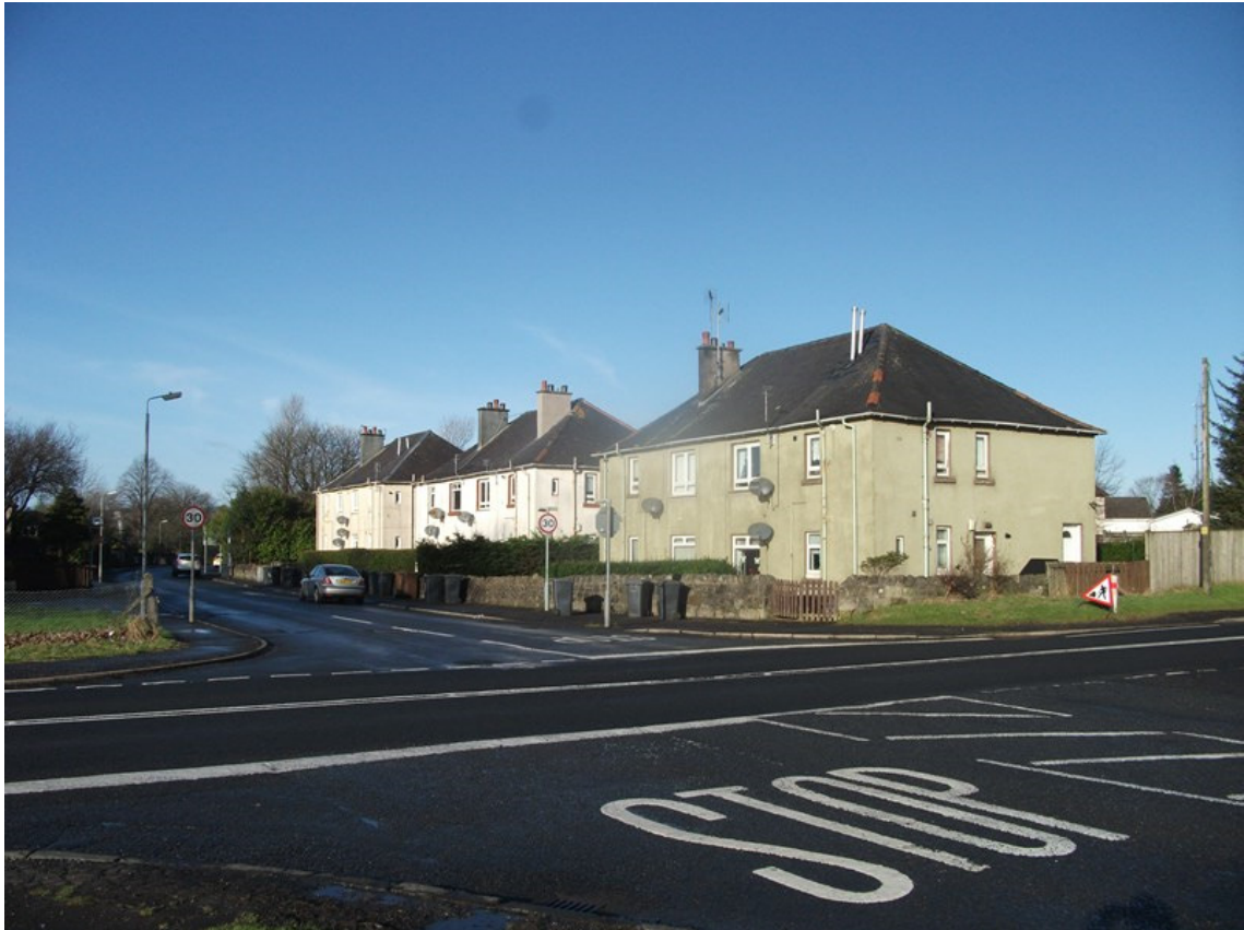
Photograph 8:24: View of Wardrop Terrace looking northwest
