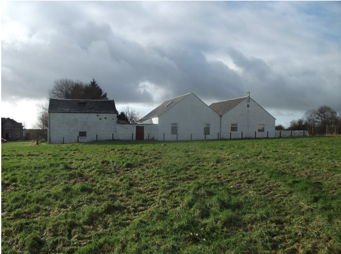
Photograph 8:11: View of 16 Barrmill Road looking southwest
