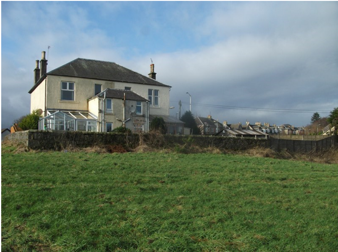
Photograph 8:10: View of 12 and 14 Barrmill Road looking southwest
