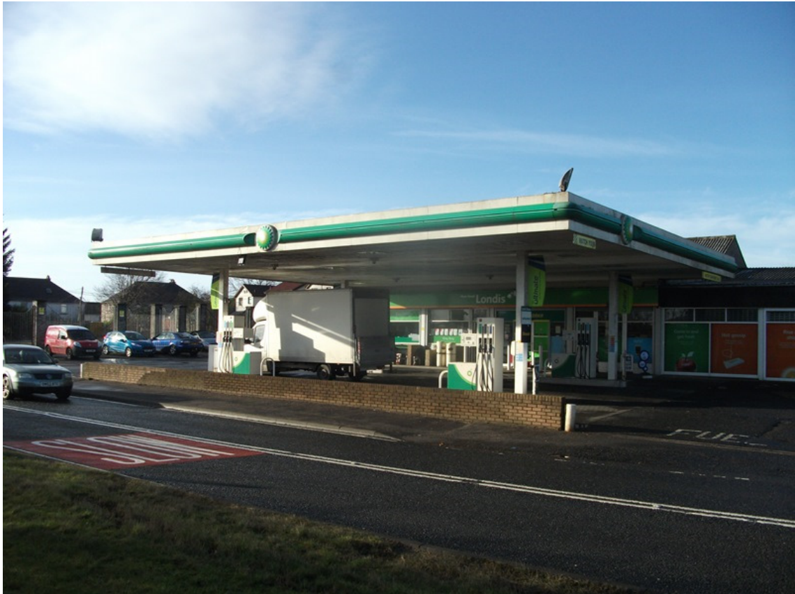
Photograph 8:26: View of Thomson of Beith looking west
