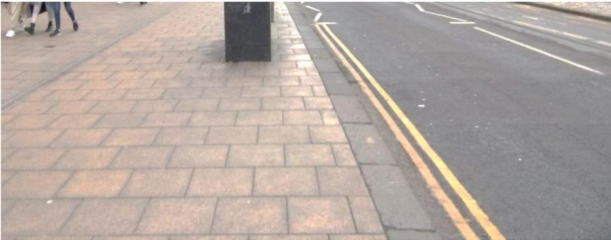
A street with a contrast value closest to zero would be Victoria Street (Figure 4-6) with a value of -0.1. The kerb on Victoria Street is made from a dark grey stone and the footway appears to be made from a similar dark grey stone slab. It is very difficult to distinguish between the footway and kerb here as they appear to be very similar in colour and darkness.
