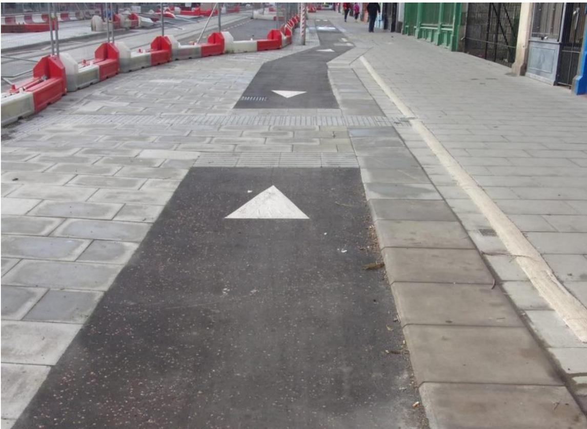
From the survey, low kerbs appear to be found in new build pedestrian busy areas, such as Leith Walk. The next lowest locations, York Place and Elder Street, are both 55mm. At York Place the kerb again separated the footway from the cycle track. On Elder Street however the kerb separated the footway from the carriageway.
