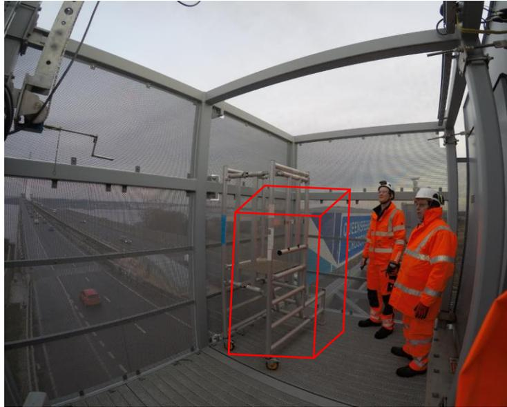
The mesh ahead of the lidar position will be removed :
