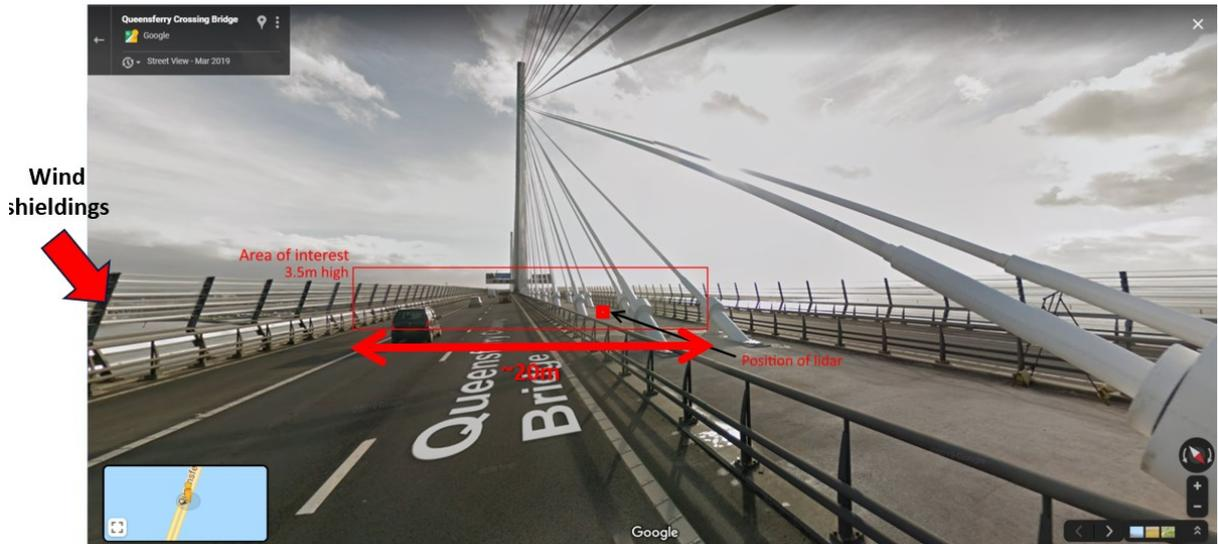
Figure 4 – Picture showing the wind shields and area of interest for the present study
