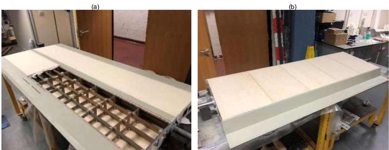
**Figure 2.7.** Pre-cut 3mm-thick plywood plates glued to the frame to close (a) the top and (b) bottom surfaces.
