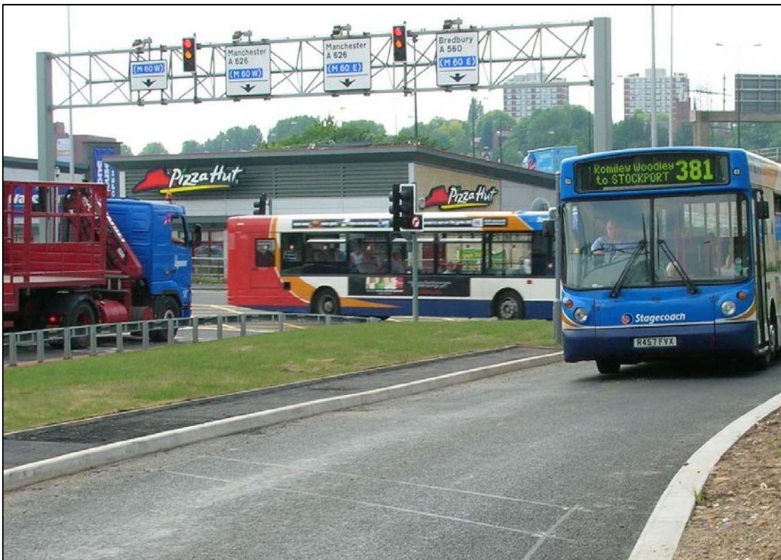
Figure G5: - An Example of a Bus Bypass at a Major Interchange
