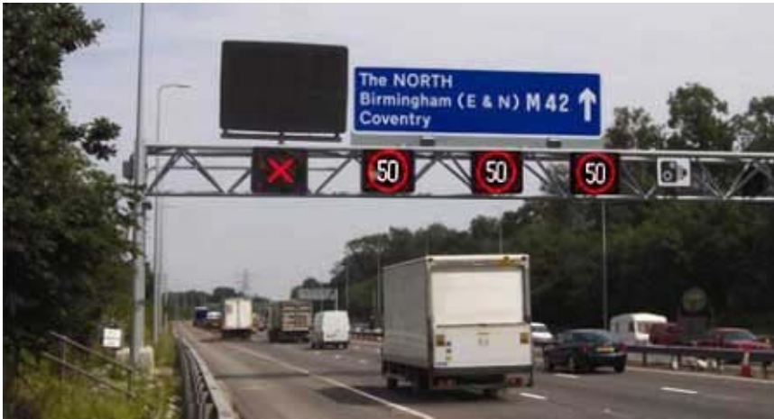
Photograph courtesy of Highways Agency
