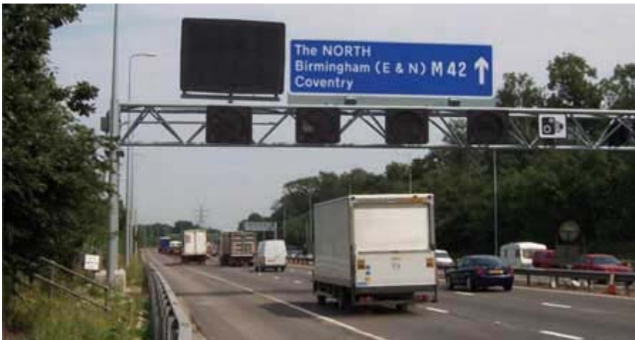
Photograph courtesy of Highways Agency
