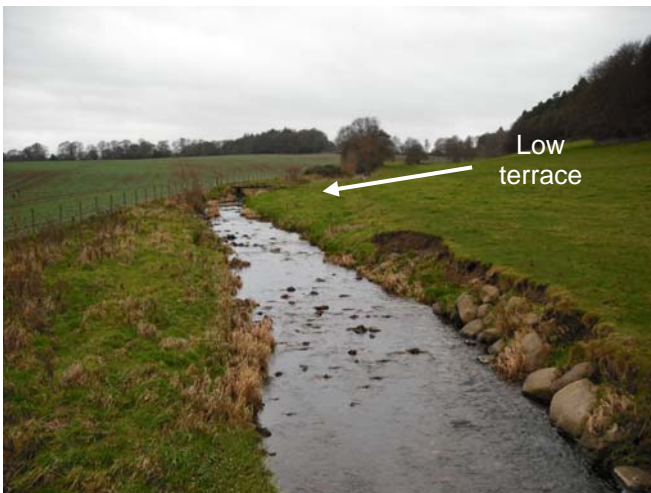
Photograph 3.6: Upstream view of Niddry Burn illustrating local erosion and protection
