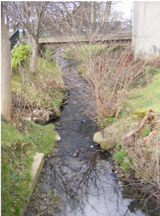
Photograph 3.10: An open channel section of Ferry Burn
