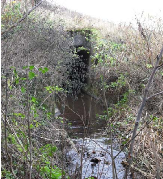
Photograph 3.4: Upstream view of the tributary of Swine Burn culvert under M9
