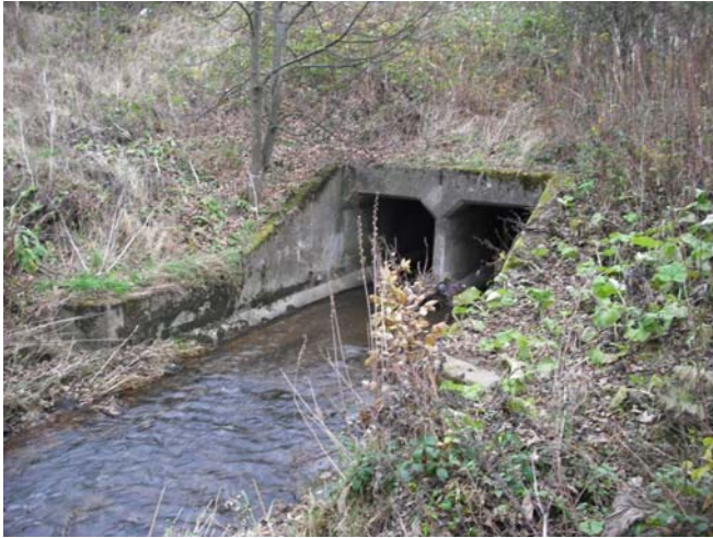
Photograph 3.5: Existing culvert on Niddry Burn
