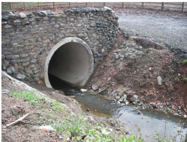
Photograph 3.9: Recent culverting of the Dolphington Burn
