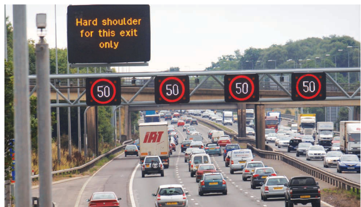
Figure 1.7: Use of Intelligent Transport Systems on the M42 in England (photograph courtesy of Highways Agency)
