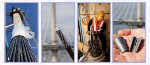
high density polyethylene (HDPE). Each strand is made up of seven high-tensile, galvanised steel wires, 5.2 millimetres in diameter (photo 2). Six of the wires, coated in wax, are wound in a helix pattern around a central "king wire" which is straight. The strands are also sheathed in an HDPE coating. Think of it this way: 7 wires = 1 strand. A bundle of strands (up to 109) = 1 cable.
