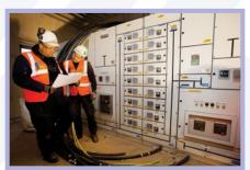
One of two main switchboards which control and distribute the power supplies to the many installations on the bridge requiring electricity.
