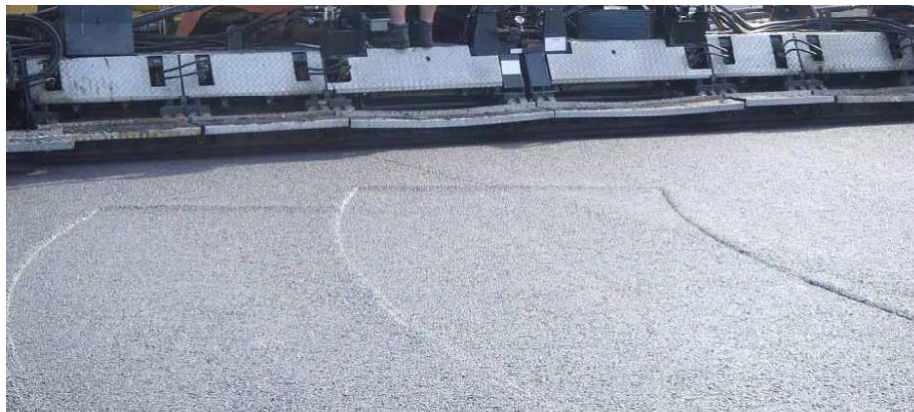
Figure NG 2.4: Roller compaction behind paver
