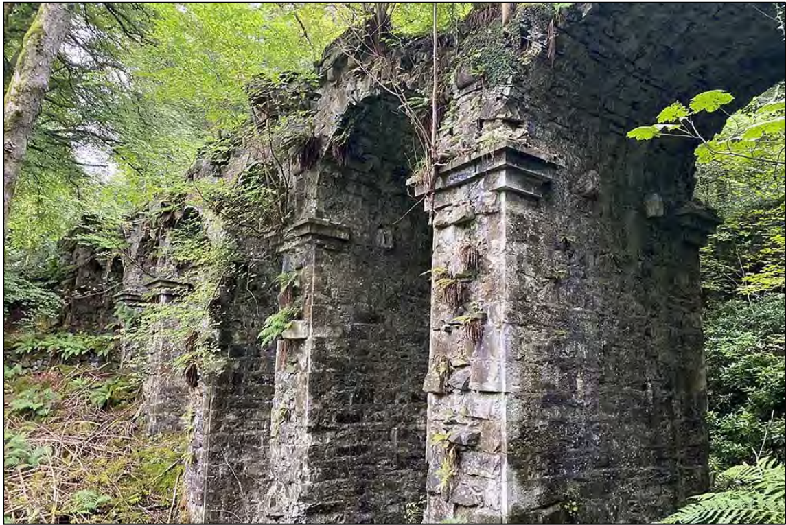
Figure 4.10: The Roman Bridge (F2.10)
