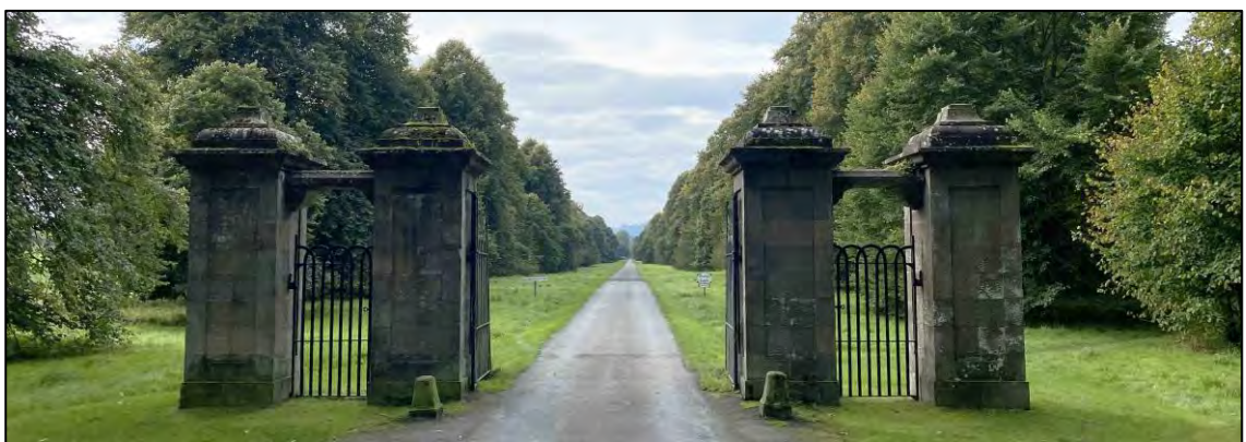
Figure 5.6: View 6 – looking west through the eastern entrance gates.
