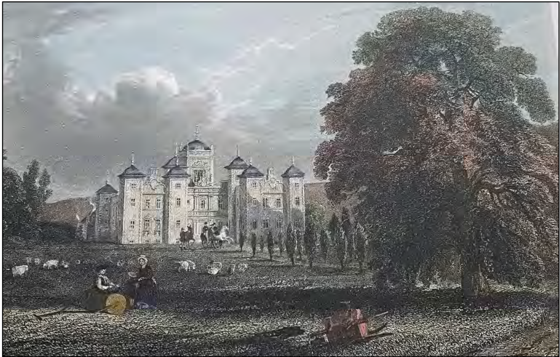
Figure 5.18: Historic View C - Looking north along the 'grand' avenue to the south of Murthly New Castle.
