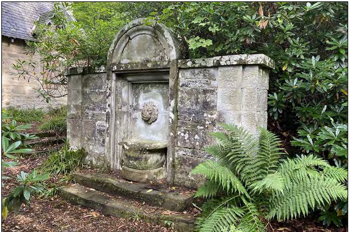
Figure 4.9: The ornamental fountain ( F2.36 ) at the East Lodge Fishing Hut
