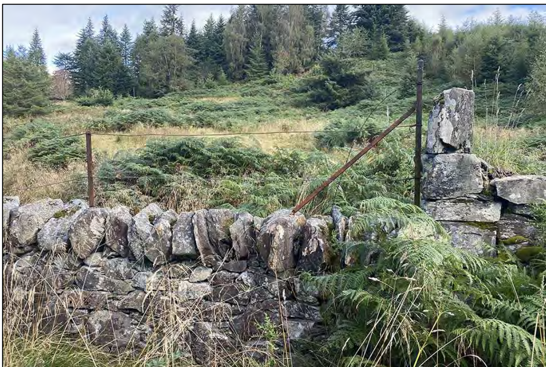
Figure 4.19: View of the boundary wall and fence to the Buffalo Park (F4.11).
