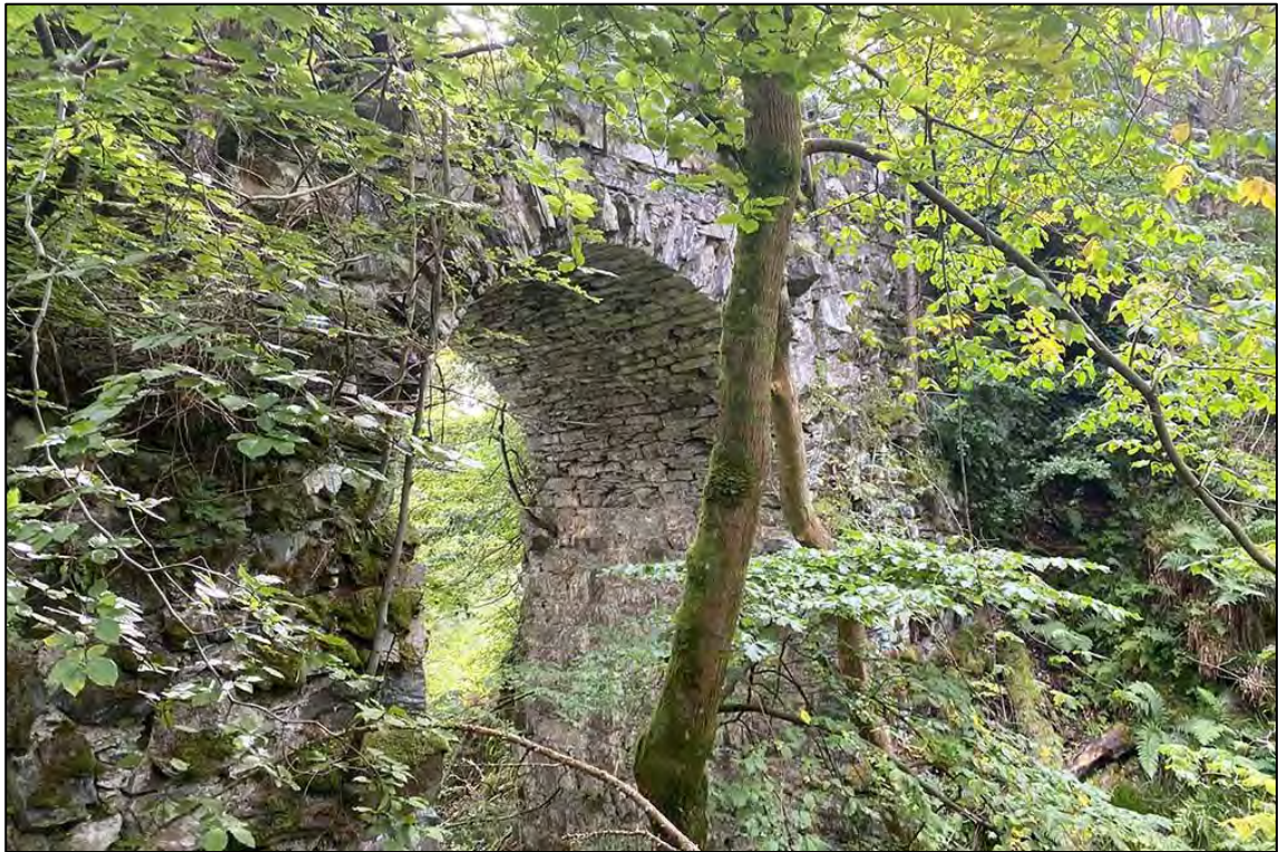
Figure 4.21: View looking up at the Stair Bridge (F4.05) from the west bank of Birnam Burn.
