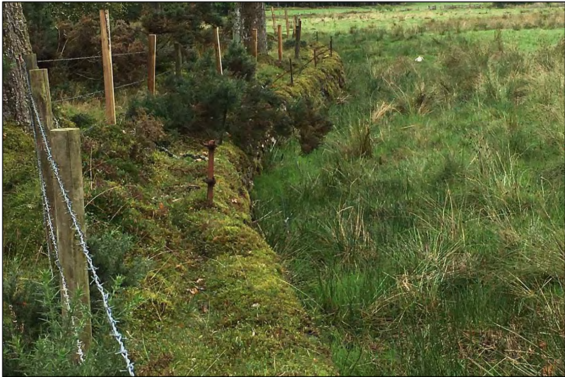
Figure 4.17: Detail of one of the sinuous curving ha-ha walls around the paddocks with the remains of metal stays, which would have supported wire fencing.
